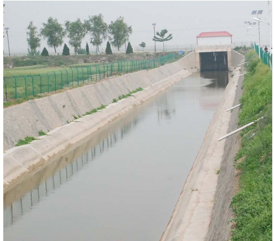
Main Channel and valve gate
