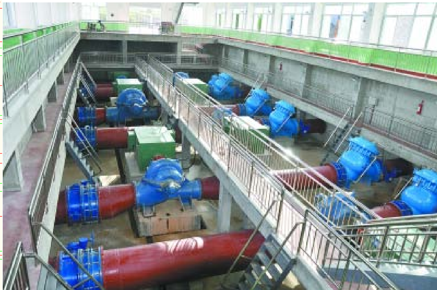
Scheme of arranging the filter, pump, check valve, hammer protection and main pipe.
