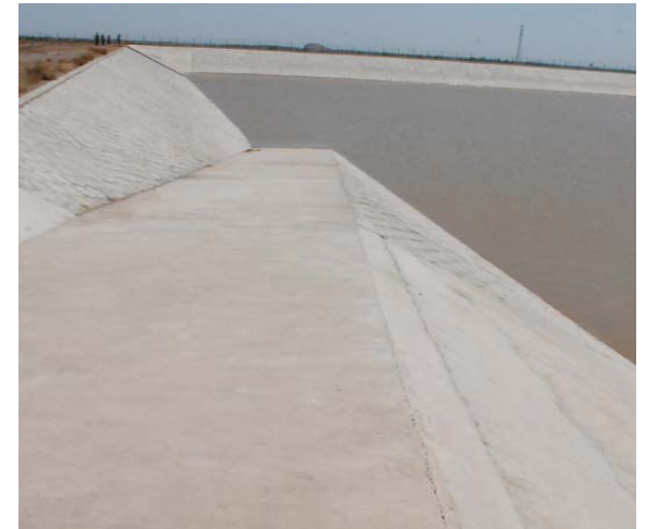
Dredging channel besides grit chamber
